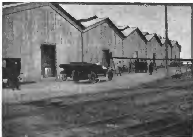
This is a gasoline storage depot at Rosario, Argentine. The gasoline is carried in 5-gal. cans, two of these cans being crated. The gasoline is brought this way from U. S. A. and stored in long rows of these warehouses instead of huge storage tanks as in U. S. A. Argentine aims at having a supply of 5,000,000 gal. of gasoline and 5,000,000 gal. of kerosene in storage all the time.
